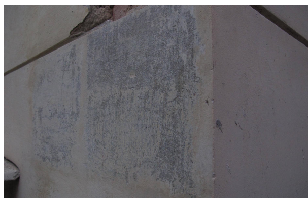
Obr. 23: Stav po provedené zkoušce – detail
